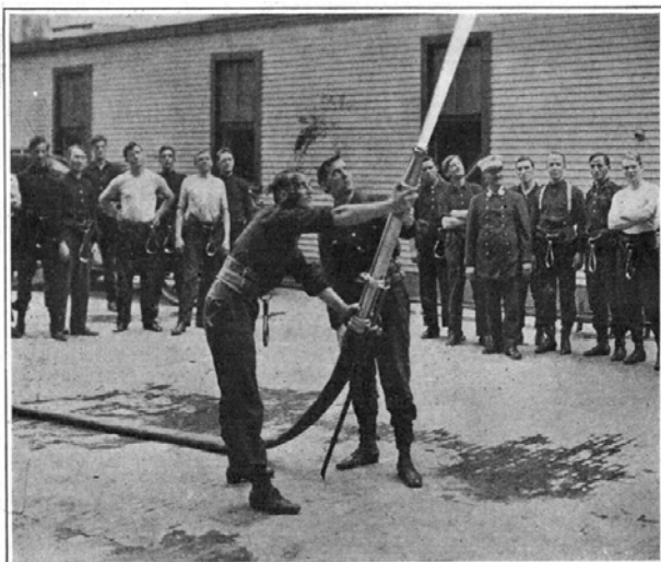
The play-pipe or deluge system. Used for a powerful stream when vast quantities of water must be poured into a burning building.
